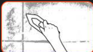
phase V: While the surface initially dries, smoothen the surface with an edge of plastic trowel.
