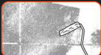
phase IV: Apply the second layer upon moistened surface.
